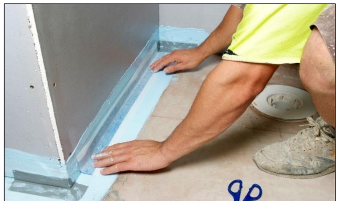
Installing Elastoproof B50 Bond Breaker Joint Band
