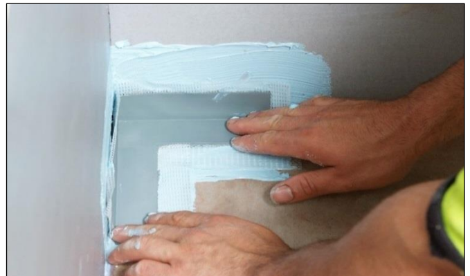
Installing Elastoproof Prefabricated Corners
