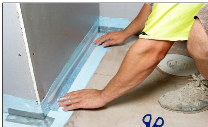
Installing Elastoproof B50 Bond Breaker Joint Band
