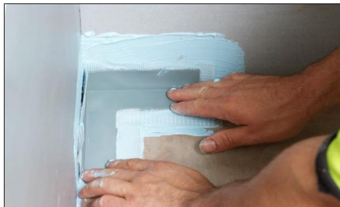
Installing Elastoproof Prefabricated Corners
