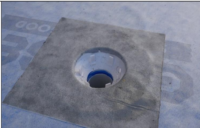
Elastoproof Butyl Square over leak control flange
