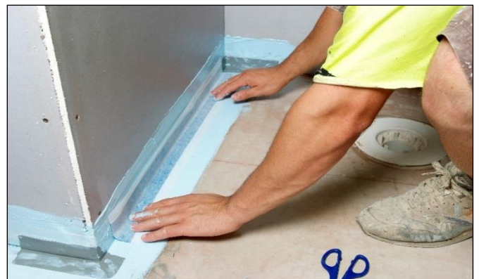
Installing Elastoproof B50 Bond Breaker Joint Band
