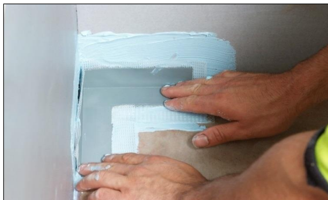
Installing Elastoproof Prefabricated Corners
