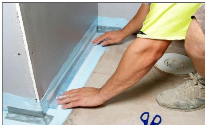
Installing Elastoproof B50 Bond Breaker Joint Band
