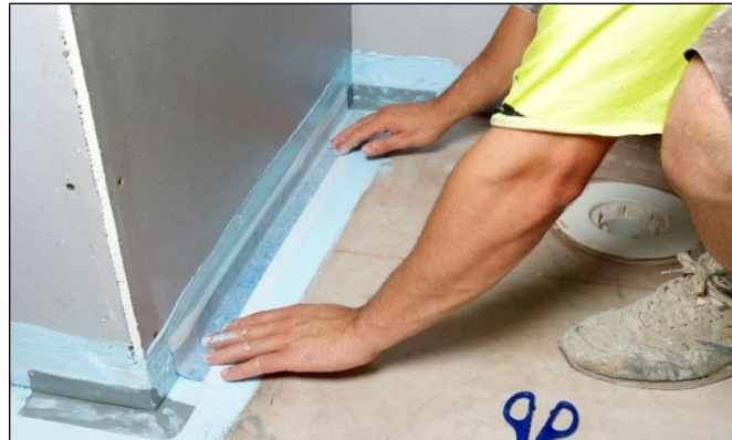
Installing Elastoproof B50 Bond Breaker Joint Band
