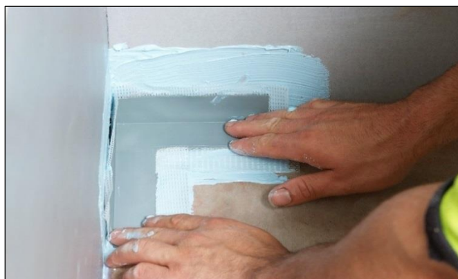
Installing Elastoproof Prefabricated Corners
