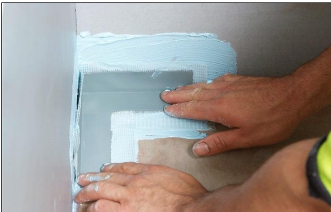
Installing Elastoproof Prefabricated Corners
