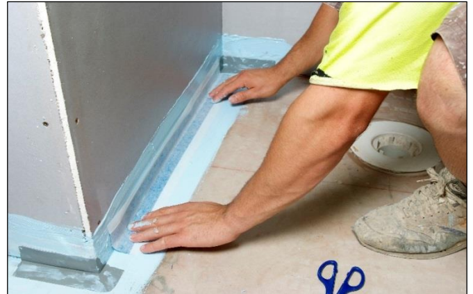
Installing Elastoproof B50 Bond Breaker Joint Band
