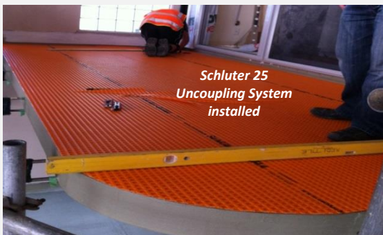
Tiled finish over Schluter 25 Uncoupling System
