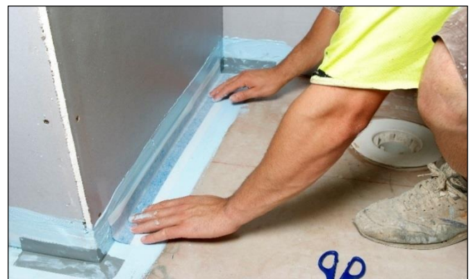
Installing Elastoproof B50 Bond Breaker Joint Band
