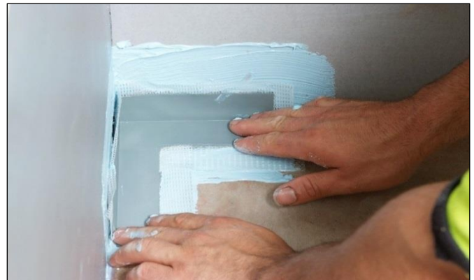
Installing Elastoproof Prefabricated Corners
