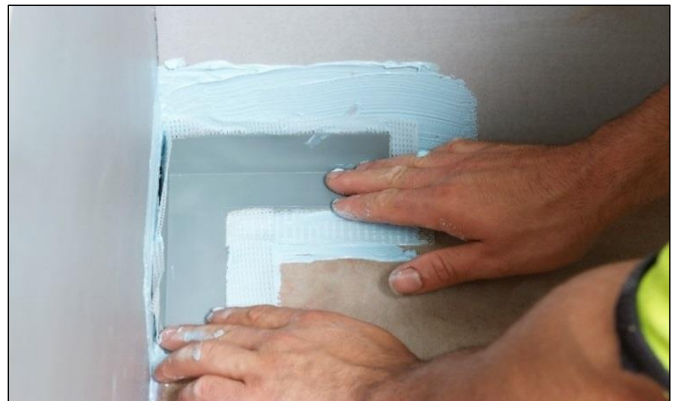
Installing Elastoproof Prefabricated Corners
