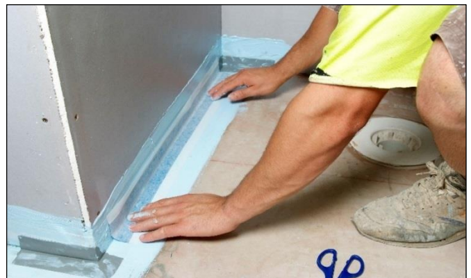
Installing Elastoproof B50 Bond Breaker Joint Band
